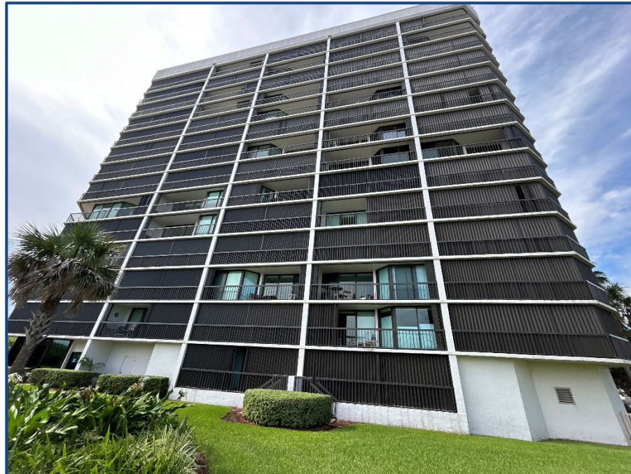
Photograph No. 2: Northern Elevation.
