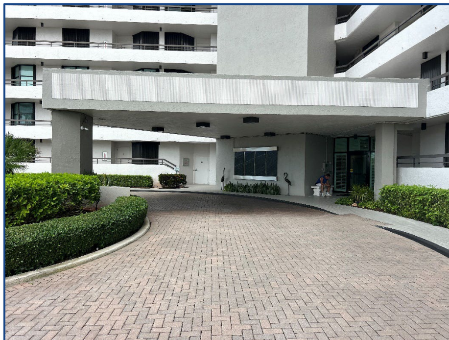
Photograph No. 6: Porte cochere at the building entrance.
