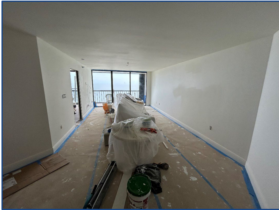
Photograph No. 33: Unit 1204 typical living room overview with work in progress.
