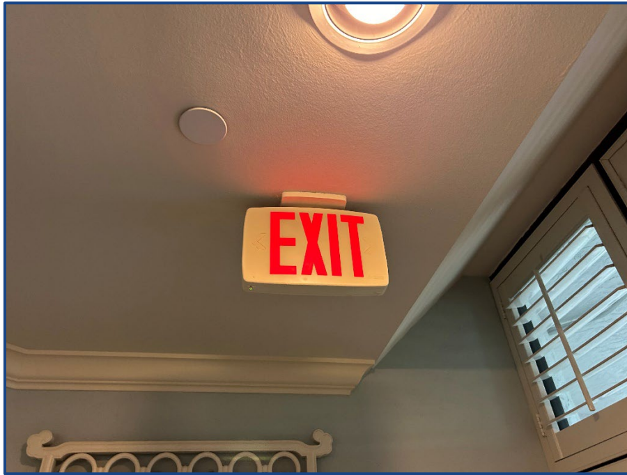
Photograph No. 18: Typical exit sign located in the first floor lobby.
