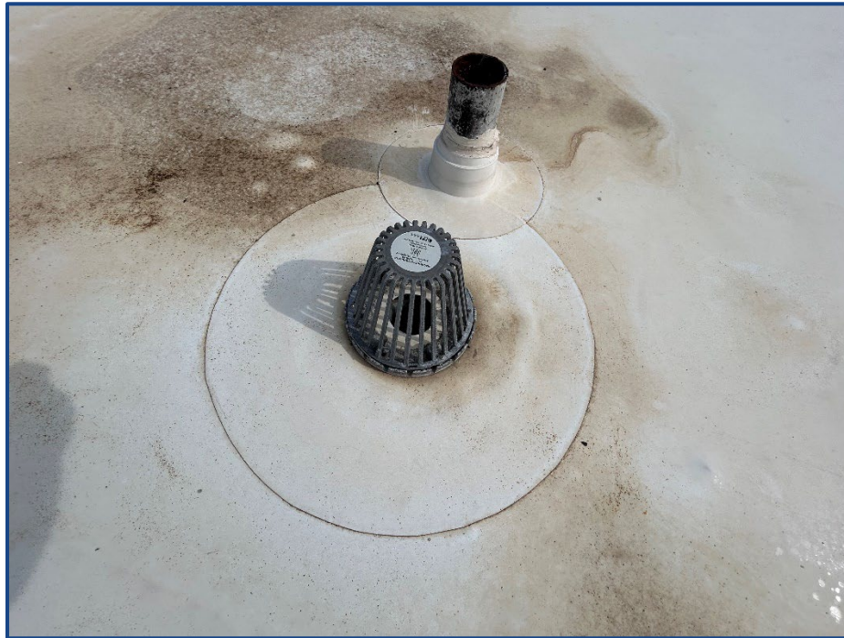
Photograph No. 16: Typical interior roof drain.
