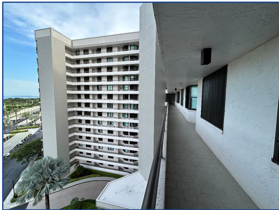
Photograph No. 10: Typical walkway at the 8th floor.
