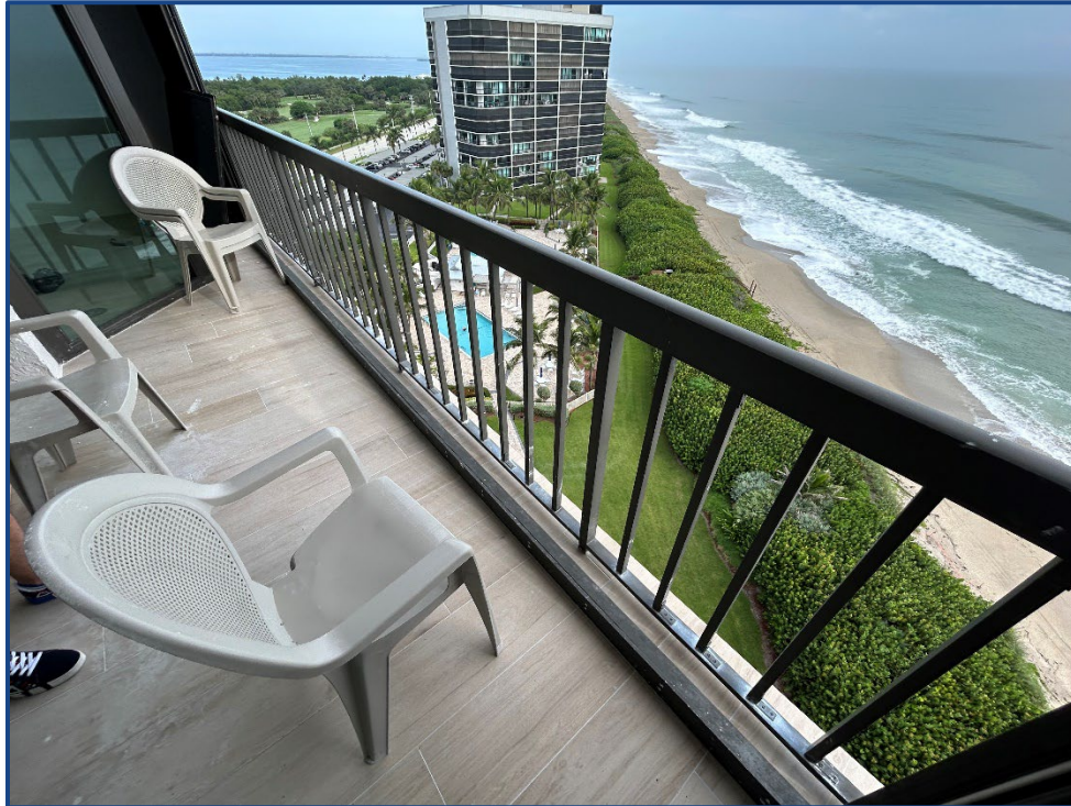
Photograph No. 34: Unit 1204 typical balcony with aluminum railings.
