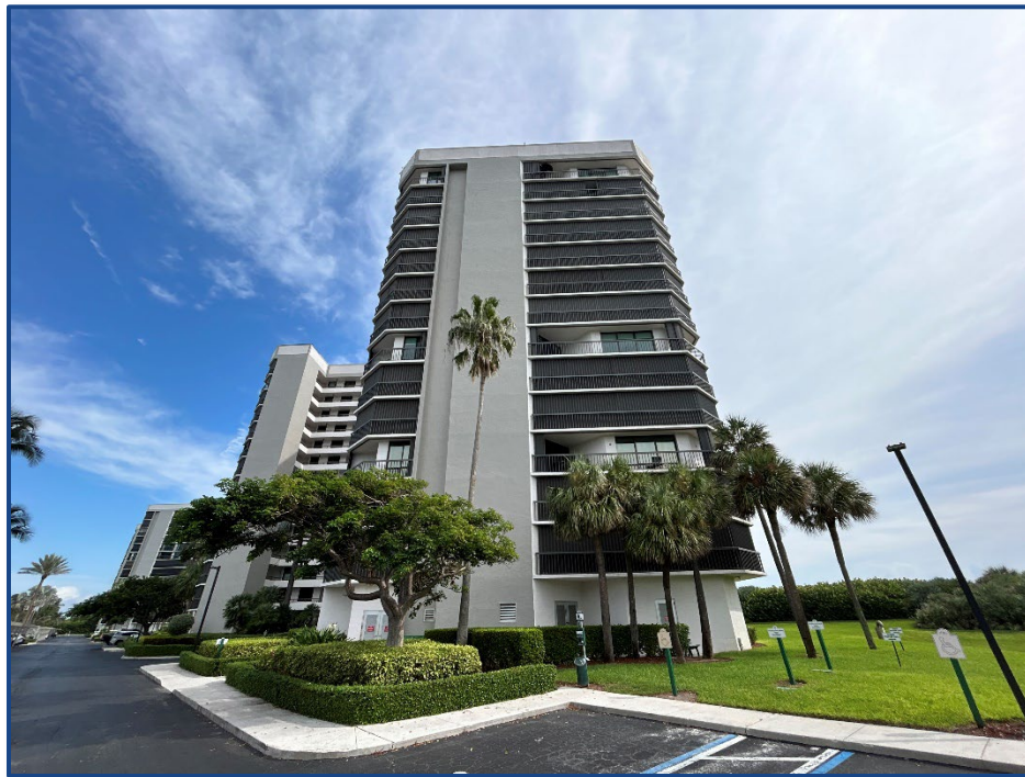
Photograph No. 4: Southern elevation.
