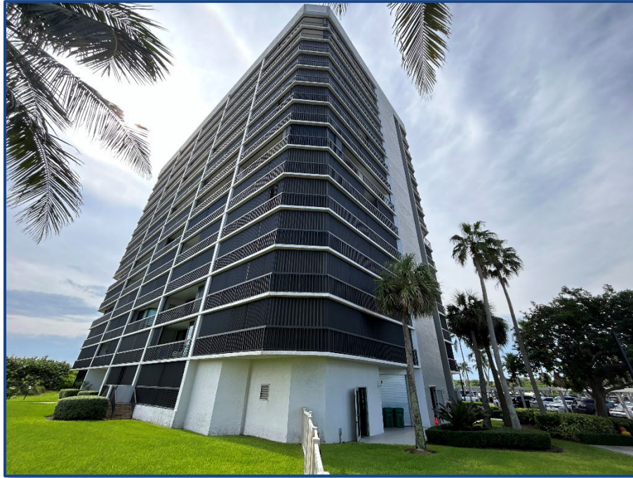
Photograph No. 3: Northern elevation.
