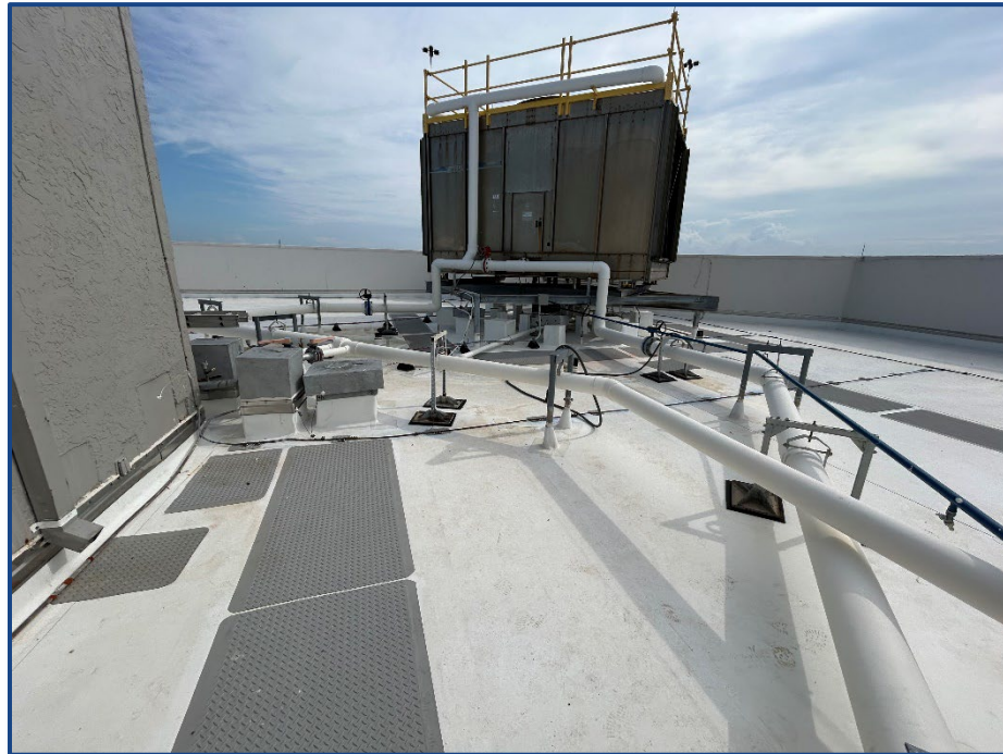
Photograph No. 13: Center of the roof with main lifted AC Unit.
