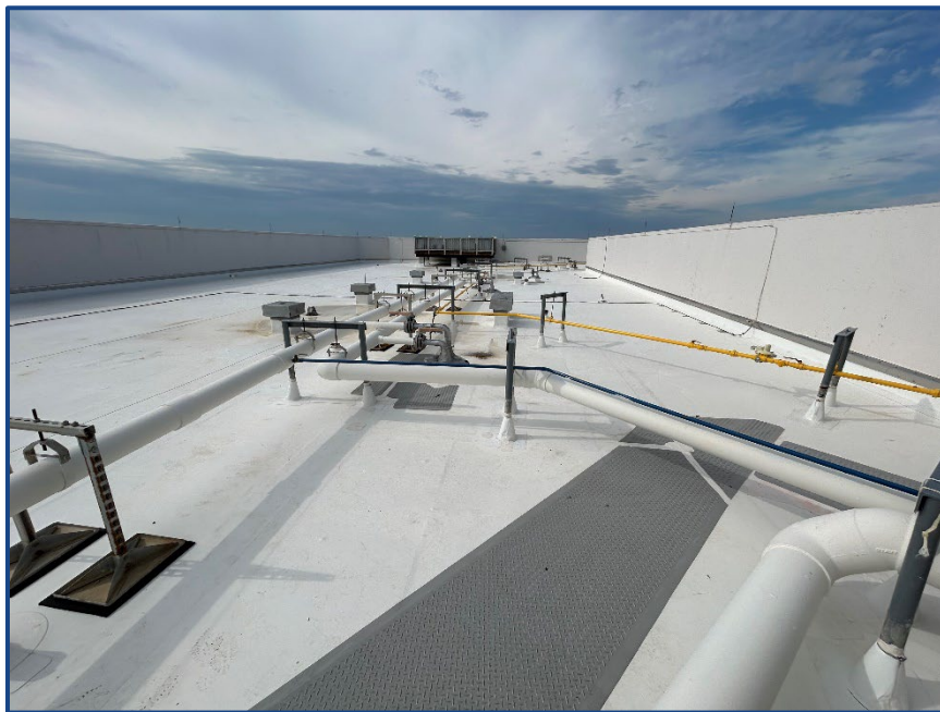
Photograph No. 12: Typical overview of the west side of the roof.
