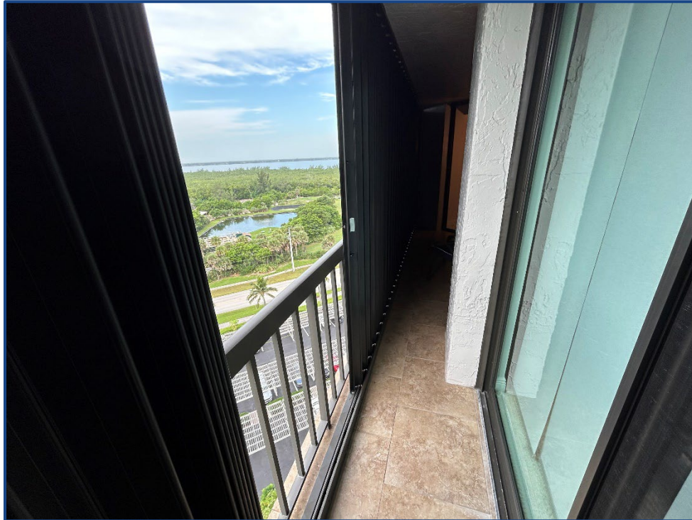
Photograph No. 30: Unit 1310 balcony area with shutters in place.
