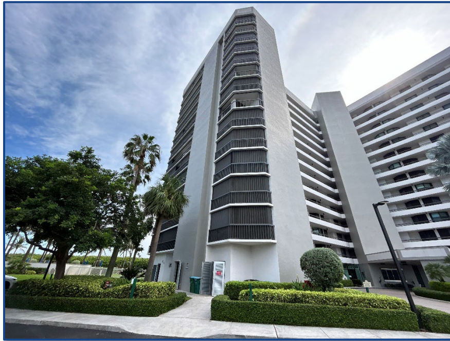
Photograph No. 5: Elevation view of the northwest corner of the building.
