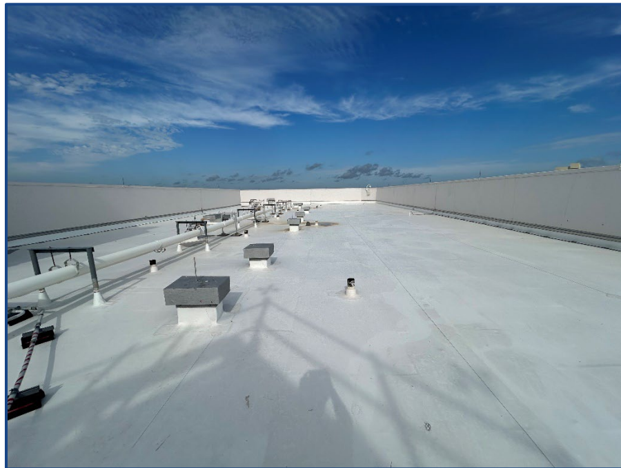
Photograph No. 14: Overview of the north section of the roof.
