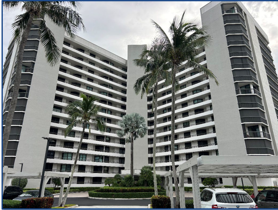
Photograph No. 1: Western elevation.
