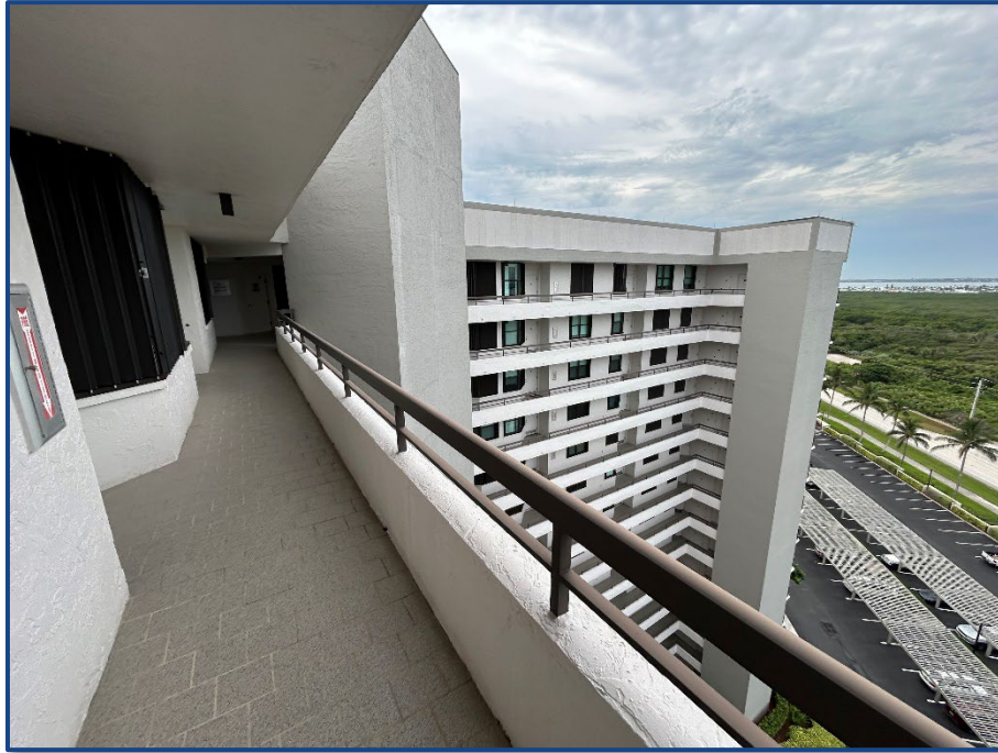
Photograph No. 9: Typical walkway at the 14th floor.
